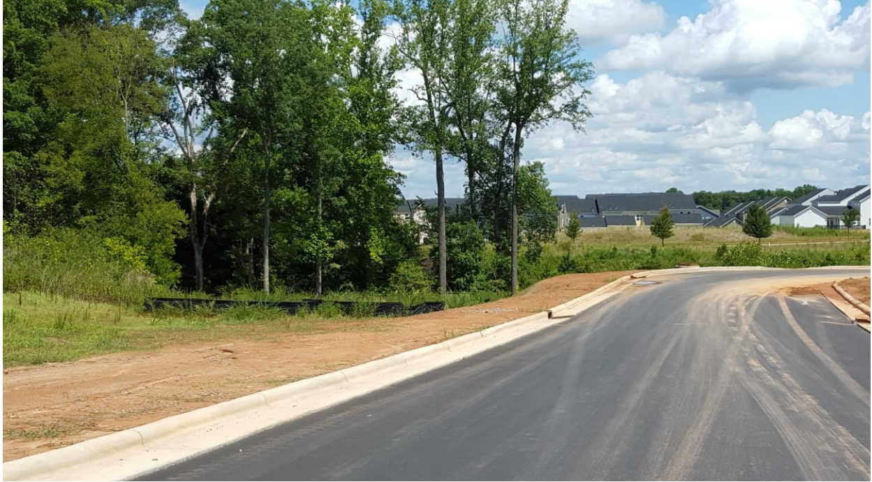
Photograph 1: Picture of start of proposed greenway trail from Zion Avenue facing towards B-1.
