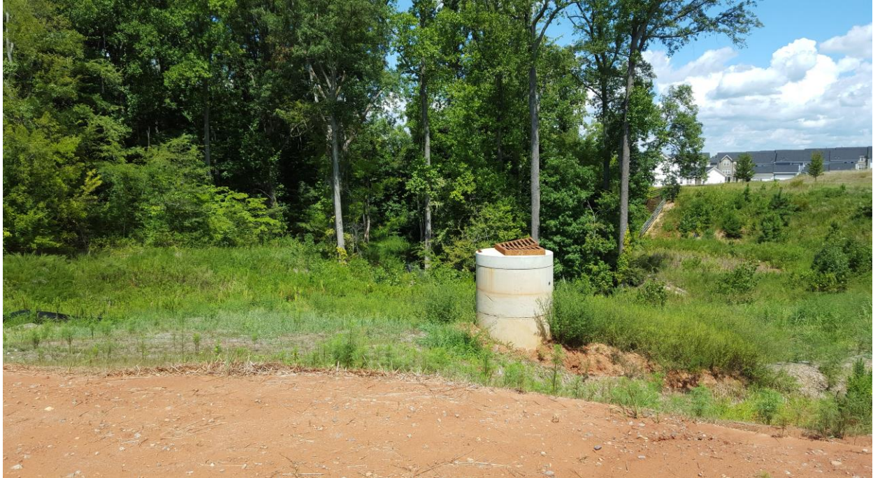
Photograph 3: Picture of start of proposed greenway trail from Zion Avenue facing towards B-1.
