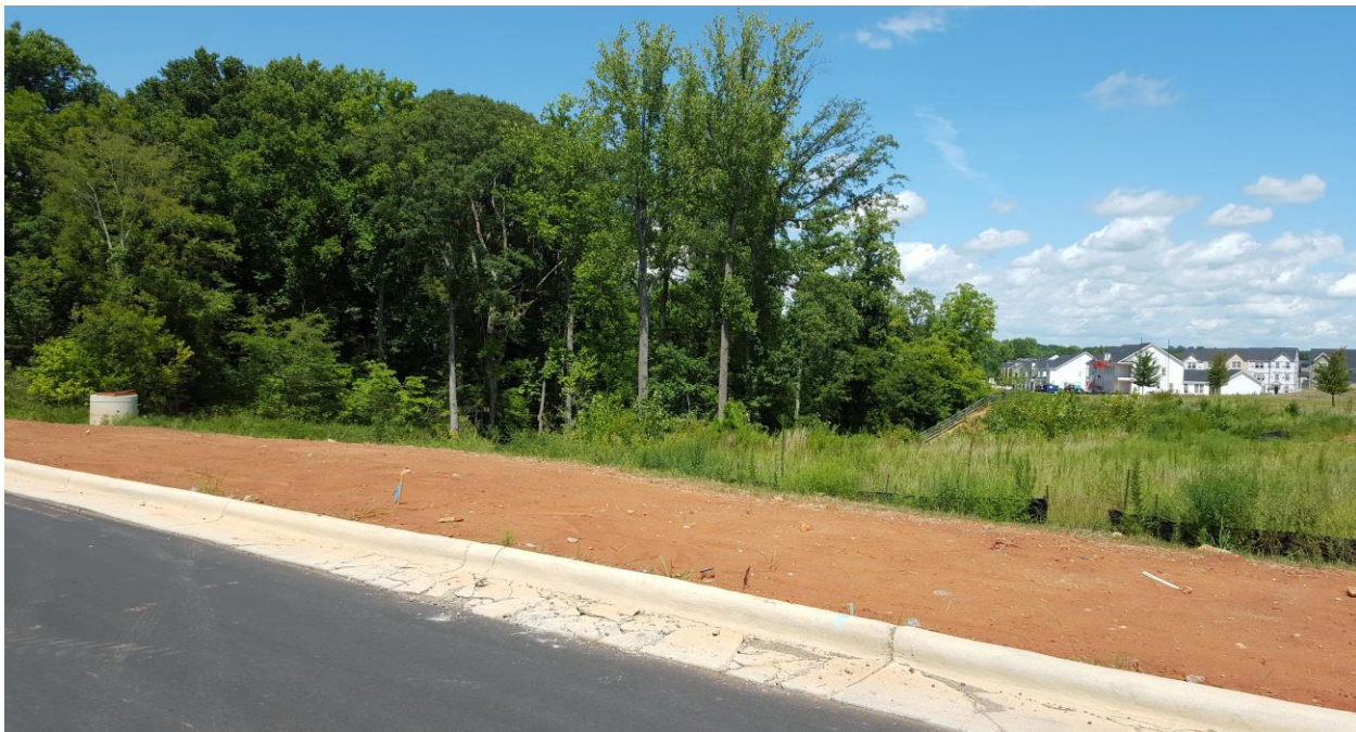
Photograph 2: Picture of start of proposed greenway trail from Zion Avenue facing towards B-1.
